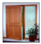
Consists of stiles, rails and one or more panels, the stiles and rails forming the frame around the panel; "stile and rail" door.
