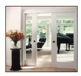
An interior French door consists of stiles, top and bottom rail and divided glass panels or lites; used as singles and pairs.
